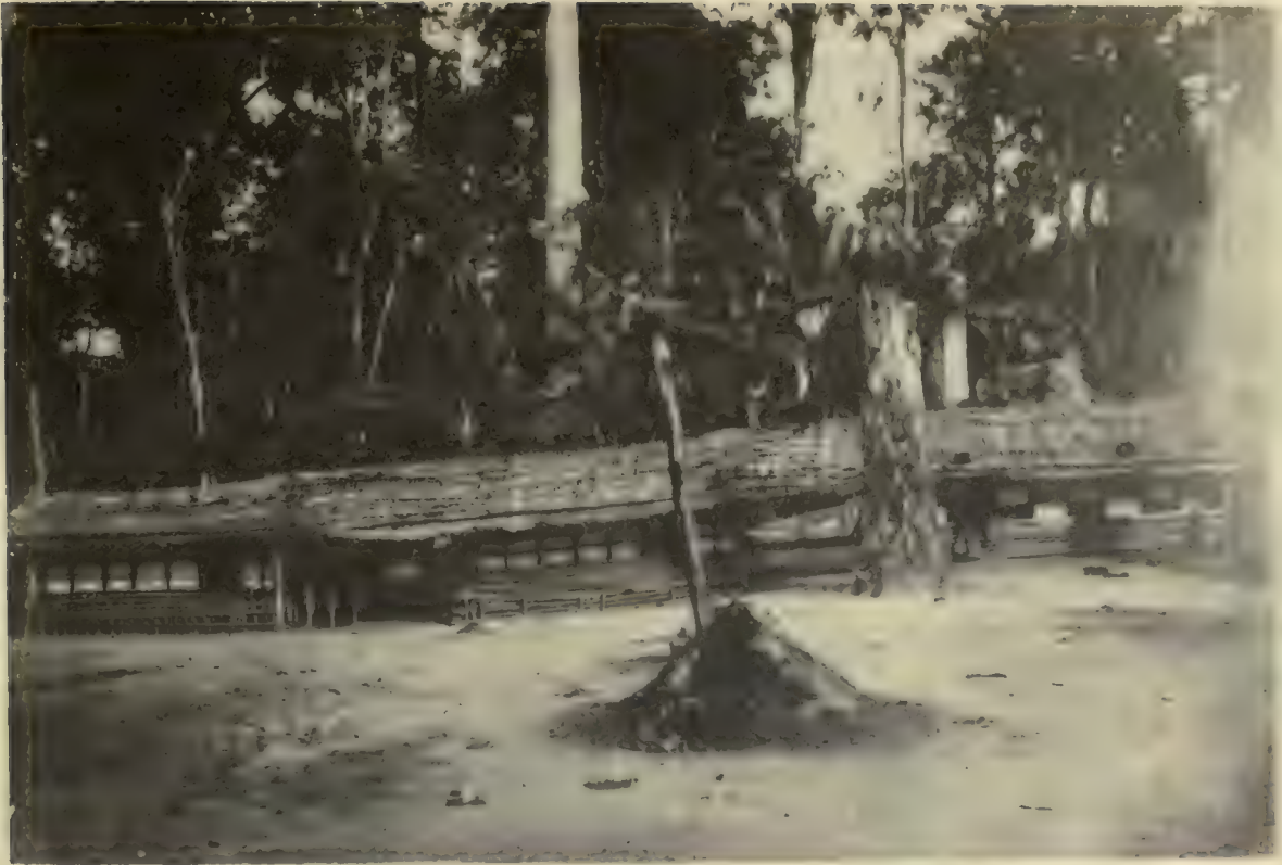
HOUSE CONSTRUCTION, FOMA.
